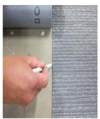
**3.** Roll/fold the first sheet. Mark the position of the joint on the subfloor.
